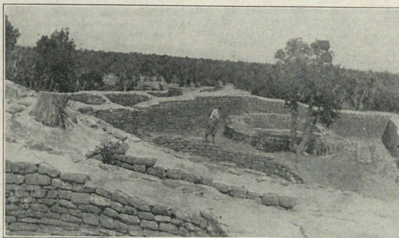
Showing the "Cells" in the Double Outer Wall.
